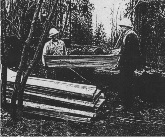
FIGURE 6. Crews worked quickly in the days after the 1962 storm in order to re-open the causeway connector to the Lions Gate Bridge and other park roadways. Images of logging crews in Stanley Park startled observers, who were unaccustomed to witnessing human labour change the landscape of the park. Source: CVA, Photograph Collection, CVA-392-540.
